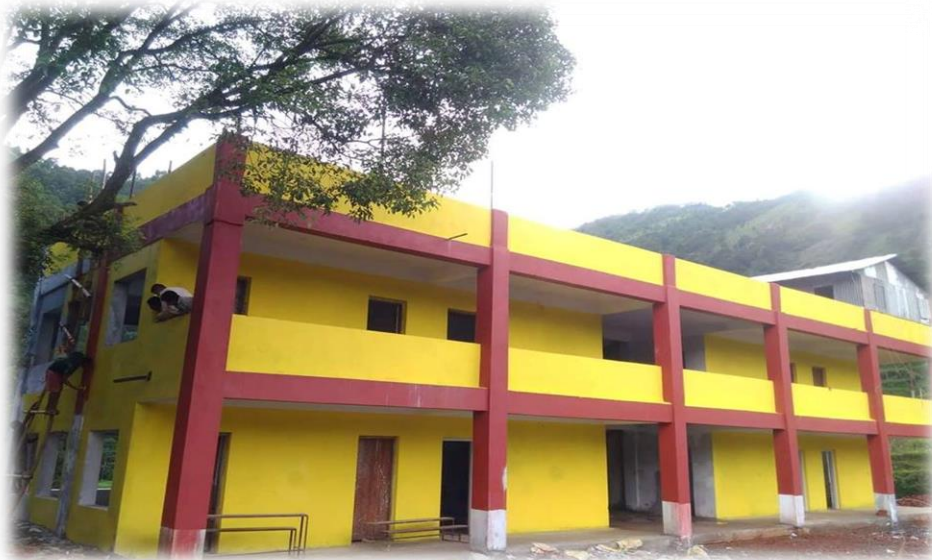
Figure 3 Kalika Lower Secondary School is in it’s final stage of completion.
